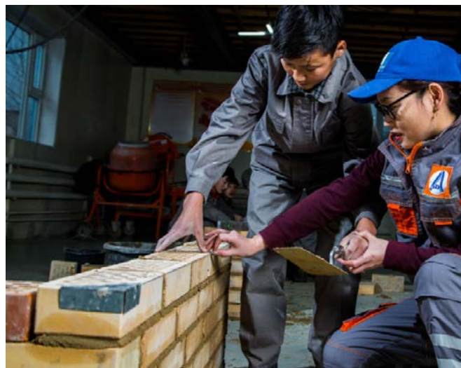
Two female builders assess the work done on a wall.
